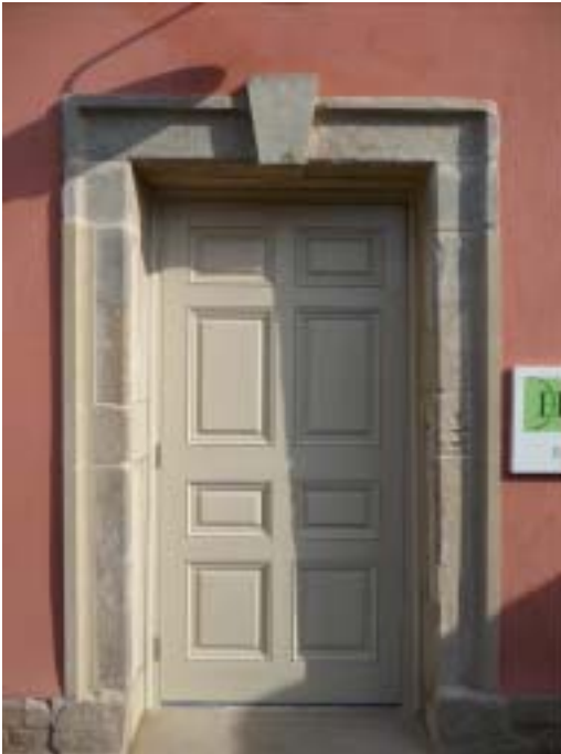
The restored original entrance
